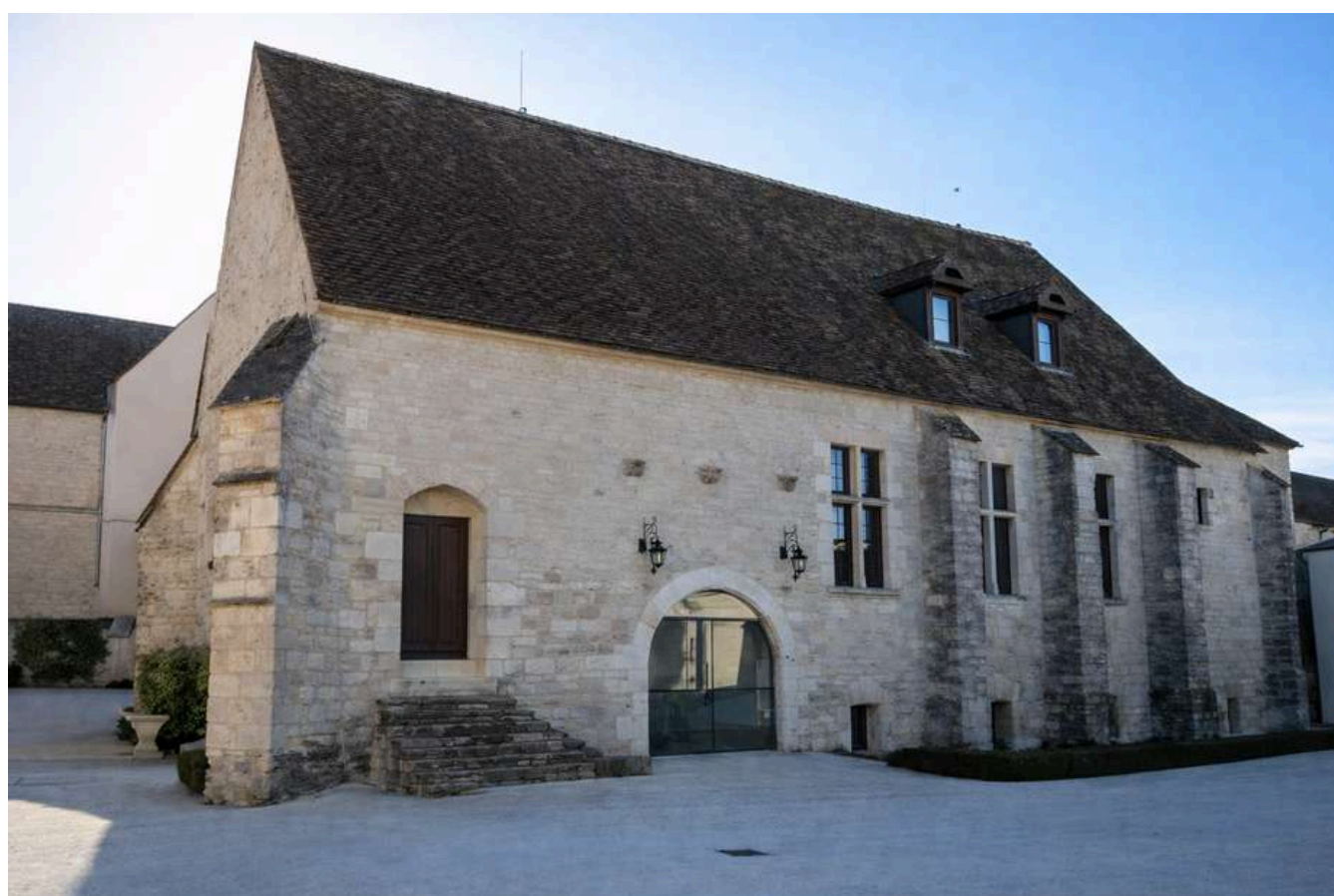
We accessed the attics via the door on the left and the cellar through the arched entrance.
